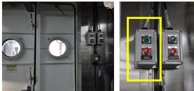
Figure 2. On/off for HPU seawater washdown is located in the wet lab near the doors to the side-sampling station.
