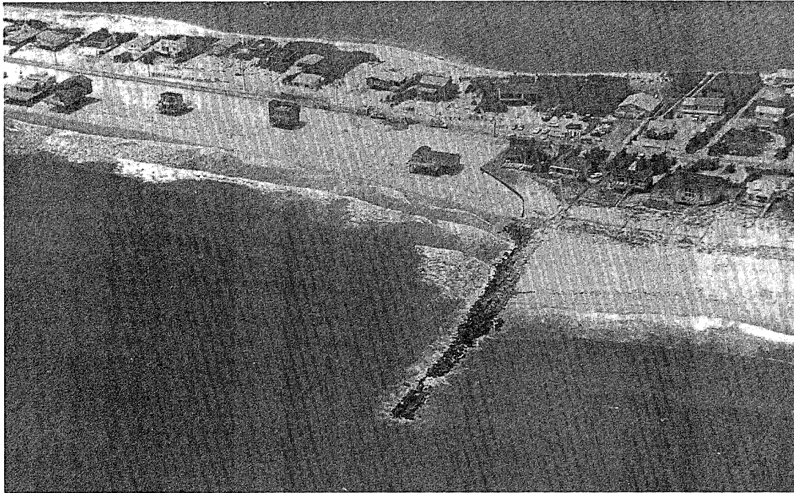
FIGURE 3-22 - Area west of the Westhampton Beach Groin Field, July 1989. Barrier at this point is only 300-500 ft. wide and has been subject to repeated washover
