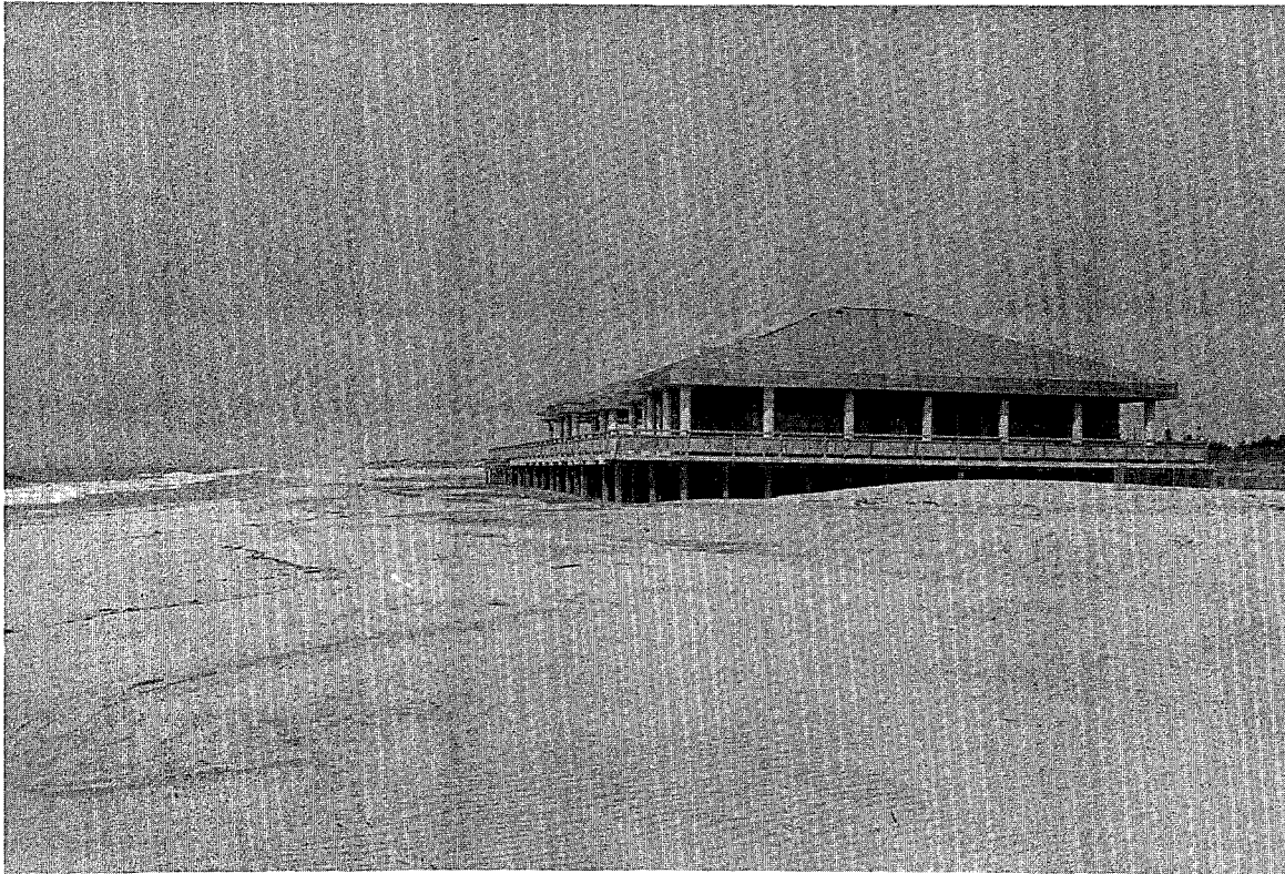
FIGURE 3-10 - Tobay Beach, May 1989. Recently reconstructed pavilion located seaward of Ocean Parkway
