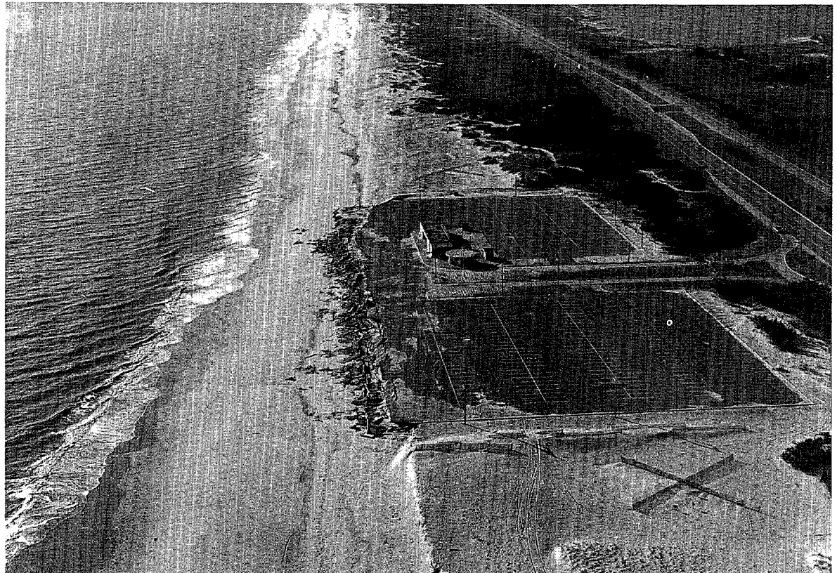
FIGURE 3-11 - Jones Beach State Park, December 1974. Erosion and subsequent abandonment of Parking Field #9 Photo courtesy of LISPC
