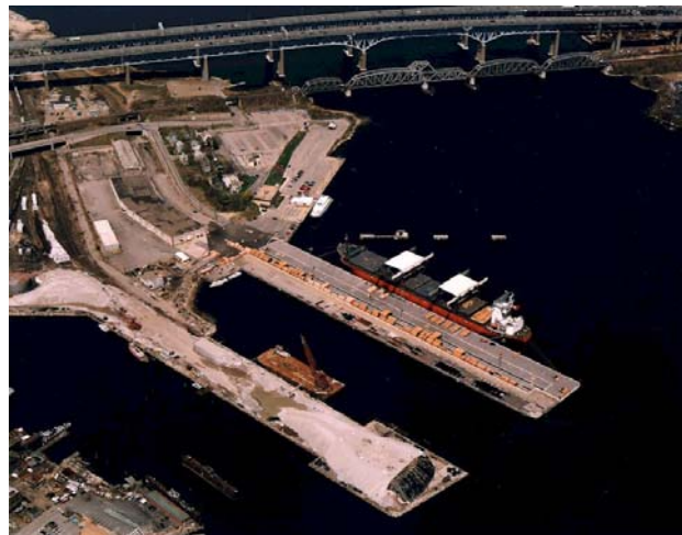
Picture Source: Connecticut Department of Transportation. 4
