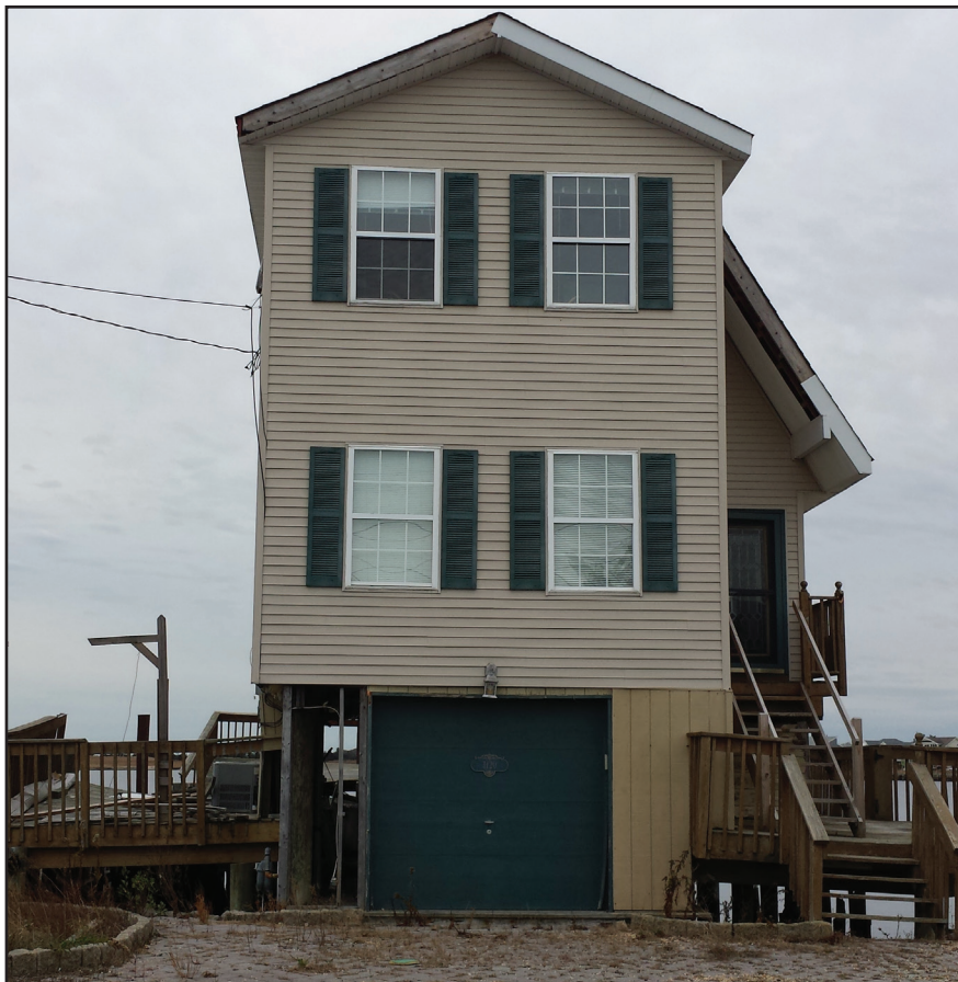
Example of raised housing for flood mitigation with incorporated storage space. Photo credit: Sarah Gonyo, NOAA.
