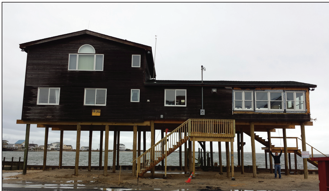
Example of raised housing for flood mitigation adjacent to the JC NERR. Photo credit: Sarah Gonyo, NOAA.
