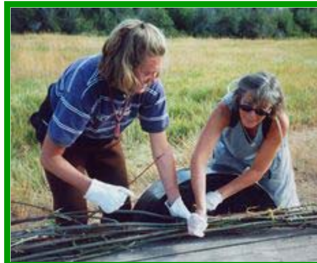
Bundling willows for bank stabilization
