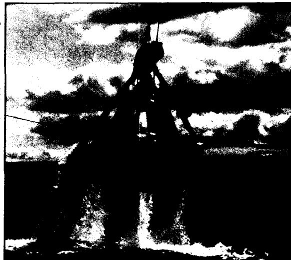
Clamshell dredge commonly used in nearshore dredging operations.
