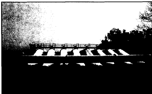
These large siphons will move fresh water and sediment from the Mississippi River to renourish and restore the productivity of the adjacent marshes.
