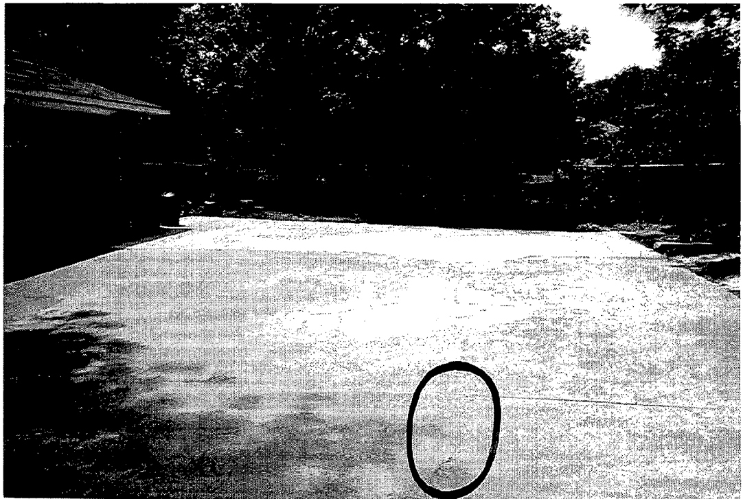
JONES CREEK-GRADE LEVEL, FENCE AND SLAB REPAIR (NORMAL TO CREEK VIEW); NOTE DAMAGE EXTENTION DISTANCE
