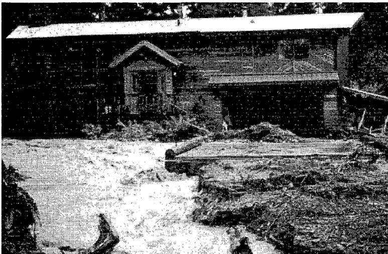
Figure 2c. Stream flowing through yard of home in Girdwood.
