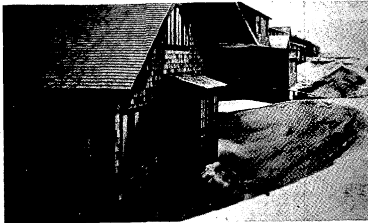
Figure 2. Blowing sand caused problems for Gearhart property owners in 1935 when sand piled up to the second floor of many residences. Removing sand, sometimes several times a year, proved expensive (from Warrenton Dune Soil and Water Conservation District, 1966).
