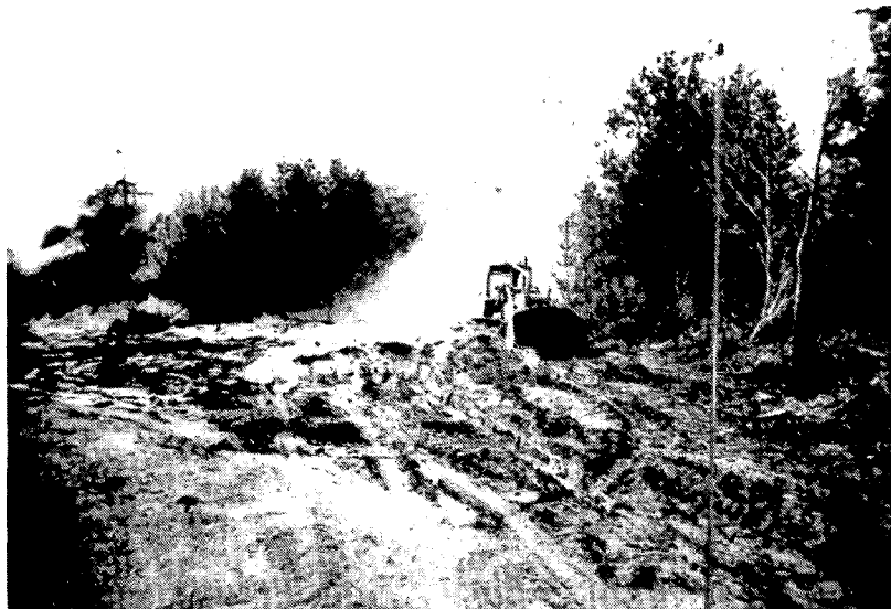
Figure 3. Sand being removed just west of Highway 101 between Glenada and Dunes City. Throughout this stretch of Highway 101, migrating dunes are within several hundred feet of the pavement.
