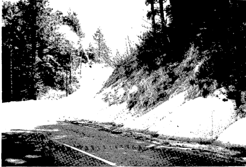
Figure 4. This migrating sand dune is constantly spilling onto the highway just north of Woods in Tillamook County.
