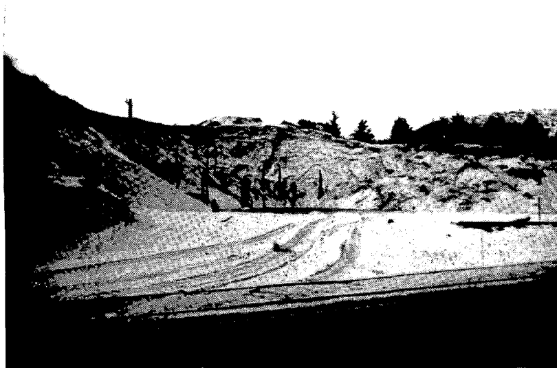
Figure 5. Sand removal activity along the Southern Pacific Railroad Line on the north slough of Coos Bay. Notice the layers of sand and the exposed trees that were buried by this in-migrating dune.
