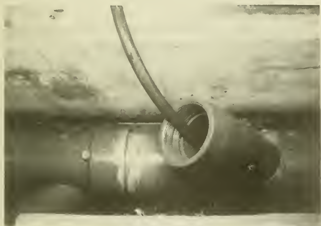
Figure 5.—Recirculating line in trench. Y fittings serve as entry points.
