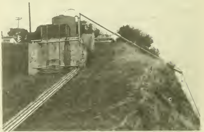
Figure 3.—Reservoir, aerator, brine tank, and pneumatic salt delivery line.
