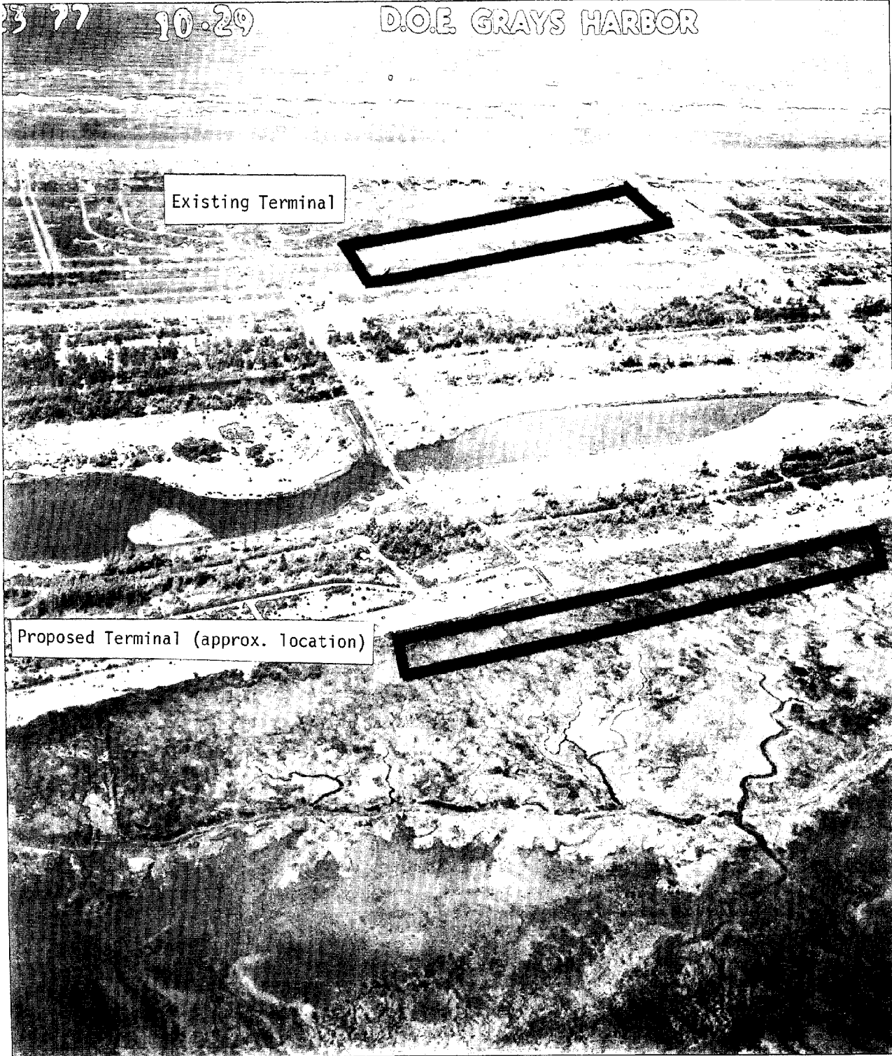
Photograph 5. Ocean Shores Existing Air Terminal and Proposed New Terminal Site.
