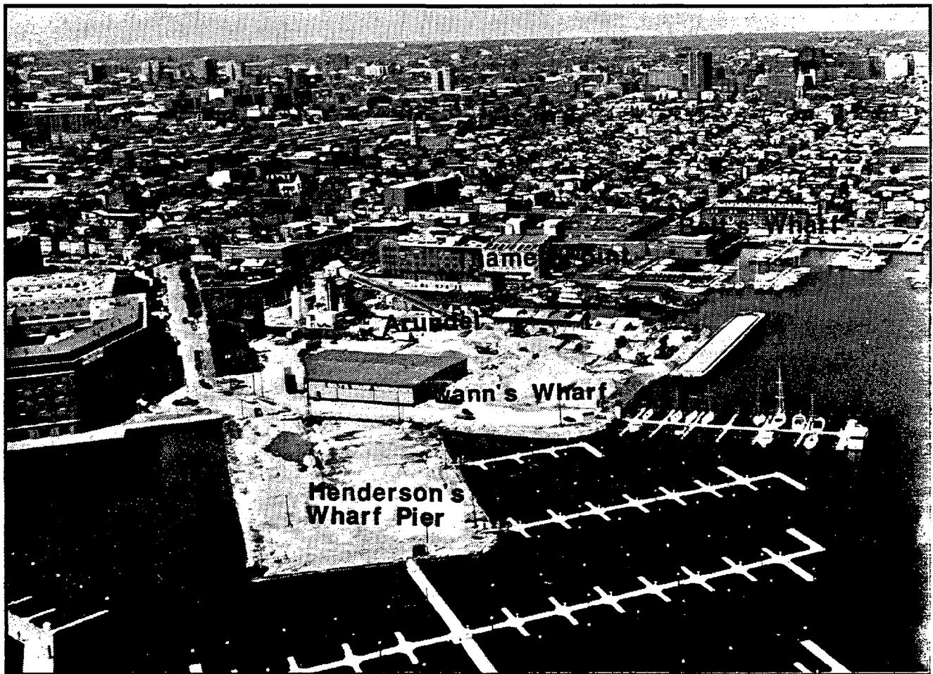
Aerial view of Henderson's Wharf, Arundel Concrete, Belt's Wharf and Thames Point
