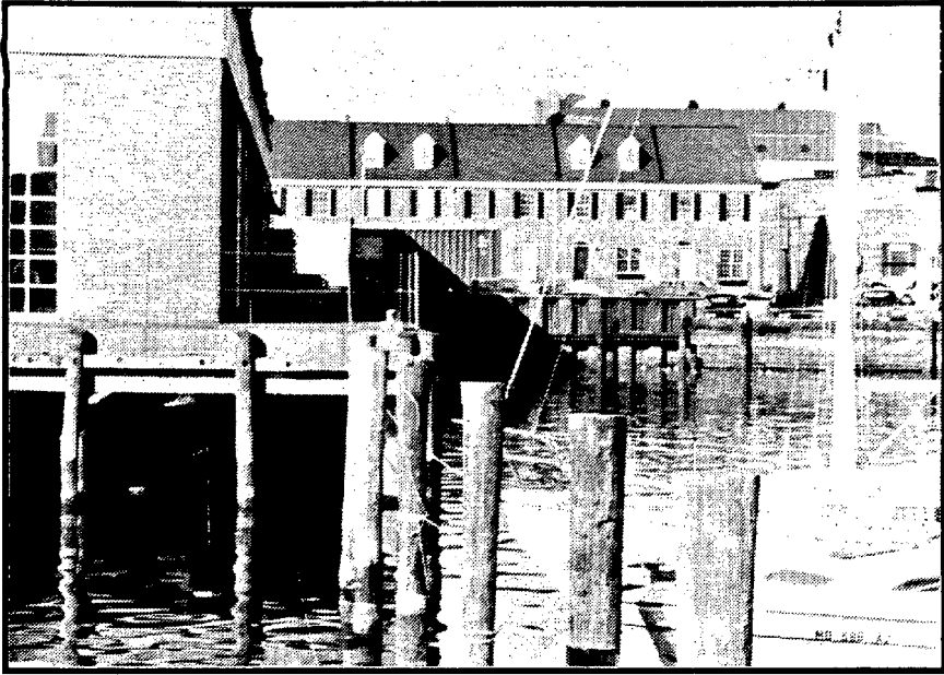
Belt's Wharf looking north
