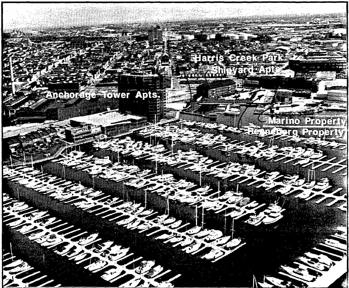
Aerial view looking northeast
