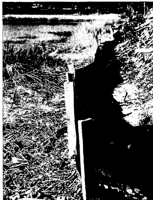
SILT FENCE PROTECTING WETLANDS
