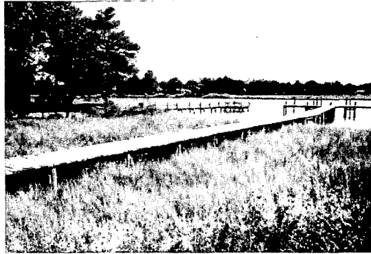
OPEN PILE PIER OVER WETLANDS
