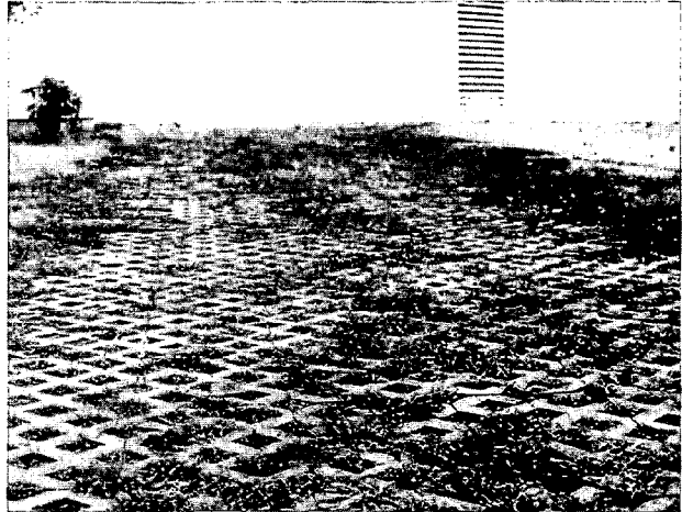
CONCRETE MODULAR PAVERS
