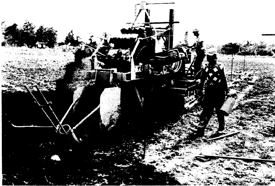
Figure 3. —Installing tile on somewhat poorly drained Lynchburg fine sandy loam. This soil is very suitable for tile drainage.
