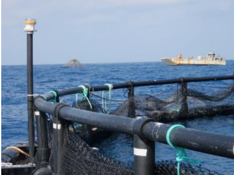
Figure 11. Photo showing handrails, stanchions, double ring configuration and navigational safety aids mounted on a float ring similar to the proposed design. The figure does not show the KikkoNet top panel, which would be mounted to the top of net pen. (Source: Kampachi Farms, 2014)
