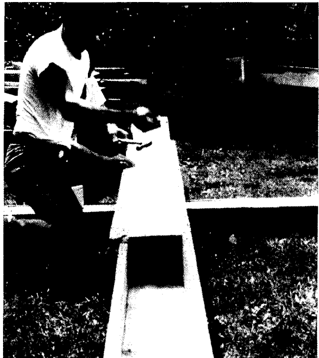
A beaver pipe allows water to pass underneath a beaver dam, preventing the flooding of nearby roads and controlling the water level. This beaver pipe was constructed and installed at Surry Mountain Lake Dam in Surry, New Hampshire.
