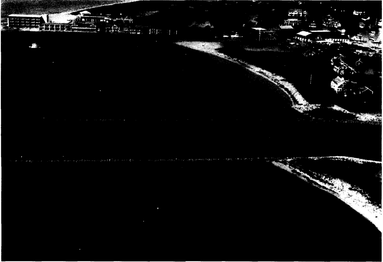
Jetties help provide safe channels for commercial and recreational vessels. The jetties at Saquatucket Harbor in Harwich, Massachusetts, also help prevent the buildup of sediment in the channel by directing and confining the tidal flow.
