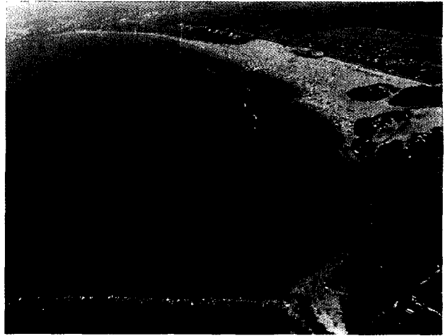
Sand Hill Cove Beach in Narragansett. The Corps constructed the five stone groins and widened one mile of the beach by the direct placement of sand.
