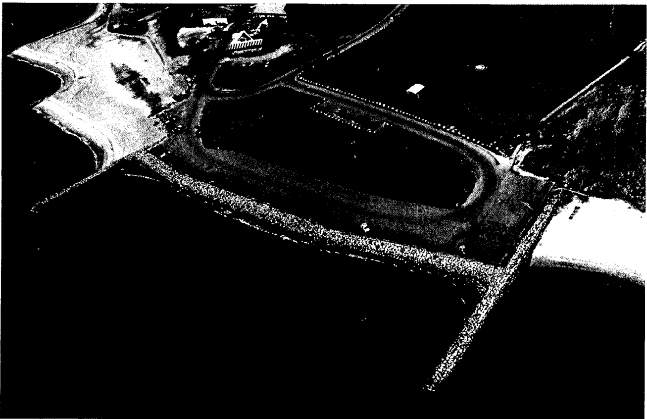
This shore protection project at Oakland Beach in Warwick, Rhode Island, is a good example of how Corps' works help protect shores and restore beaches. Sand replenishment, which widened and restored the two beach areas on the far left and far right, slows the ocean's inland advance. The four groins maintain shore alignment by trapping and retaining sand. The stone revetment, in the center of the photograph between two groins, retards erosion.
