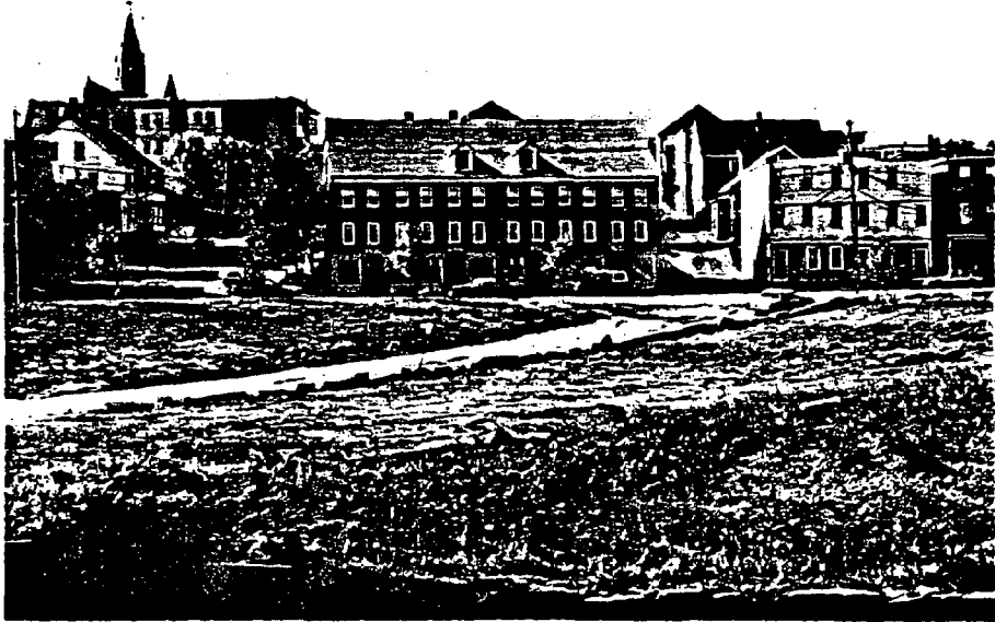
White's Wharf site and historic buildings across Water Street
