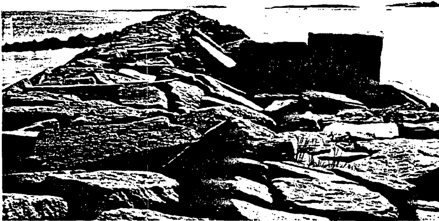
Jetties at Camp Ellis, a U. S. Army Corps of Engineers project
