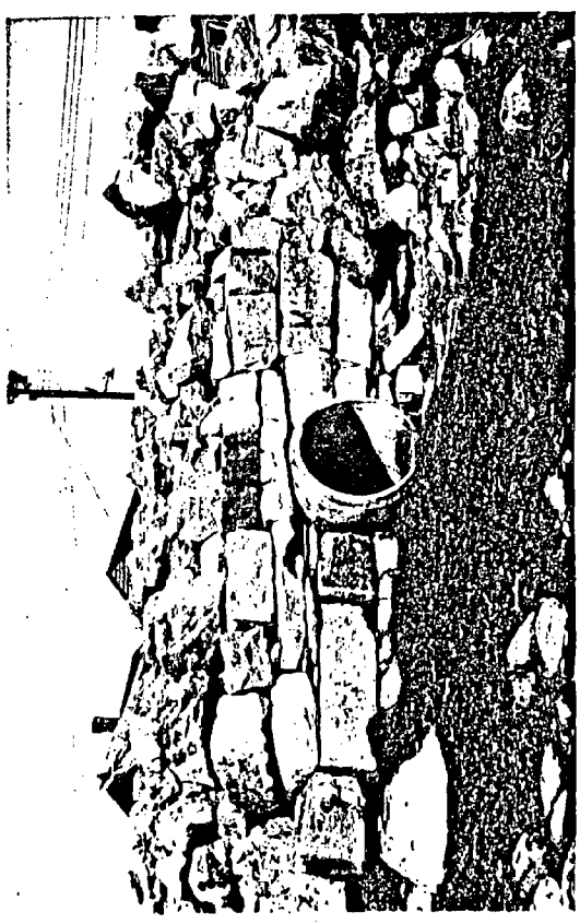
Photos of Little River Marsh and the 48" culvert installed under the fish houses in 1948. Photo at upper right shows the marsh under flood conditions. Photos from the New Hampshire Department of Public Works and Highways.
