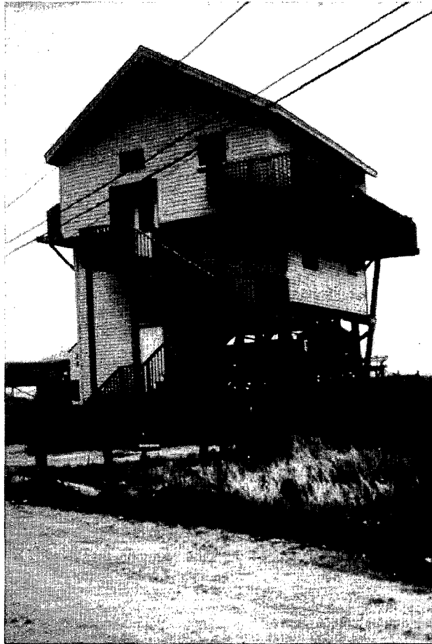
A stilt house at Misquamicut, R.I. will allow flood waters to pass underneath but in the future, with expected sea level rise, the owners may have to reach their home by boat rather than by car. (TSC Photo, 1988)
