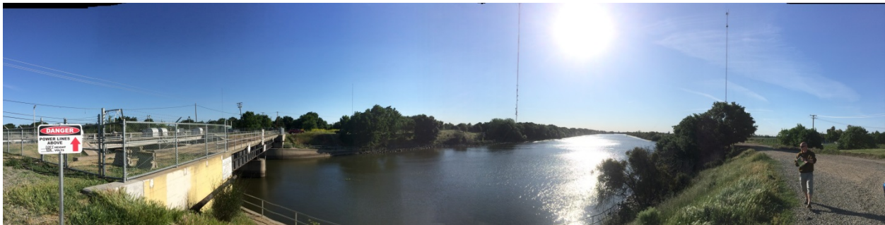
Figure 35. Picture of testing location at the west end of the Delta Cross Channel.
