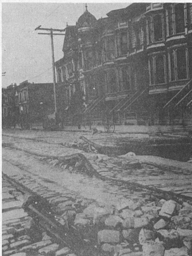
Damage to railroad tracks in San Francisco from earthquake of April 18, 1906; intensity X was assigned to this damage (see appendix 1, p. A-2).
