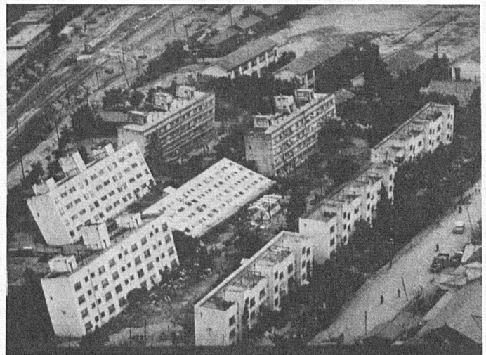
Leaning apartment houses produced by soil liquefaction during June 16, 1964, earthquake in Niigata, Japan.
