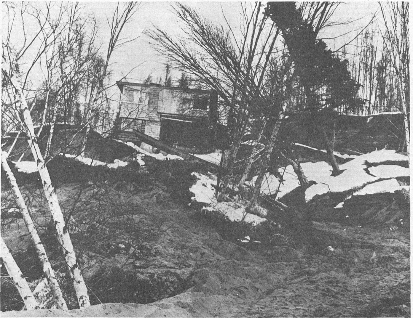
Slumping due to soil liquefaction during March 27, 1964, earthquake in Anchorage Alaska.
