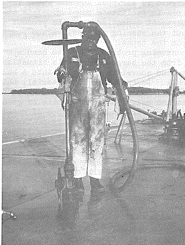
Figure 3a: Barge Washing Equipment - Butterworth Sprayers
