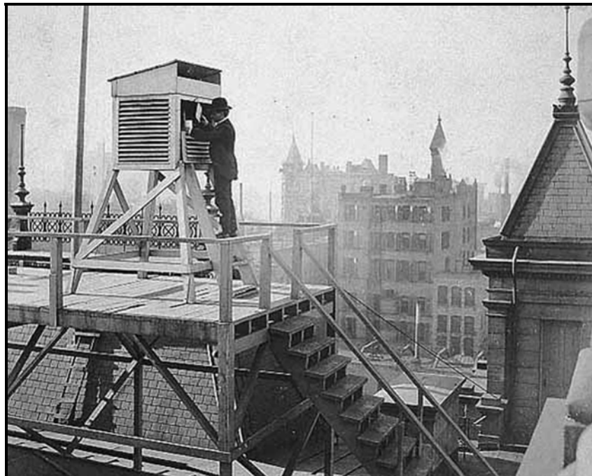
Figure 25. Instrument shelter on the roof of the U.S. Court House (circa 1890). View is southwest. From the Minnesota Historical Society.
