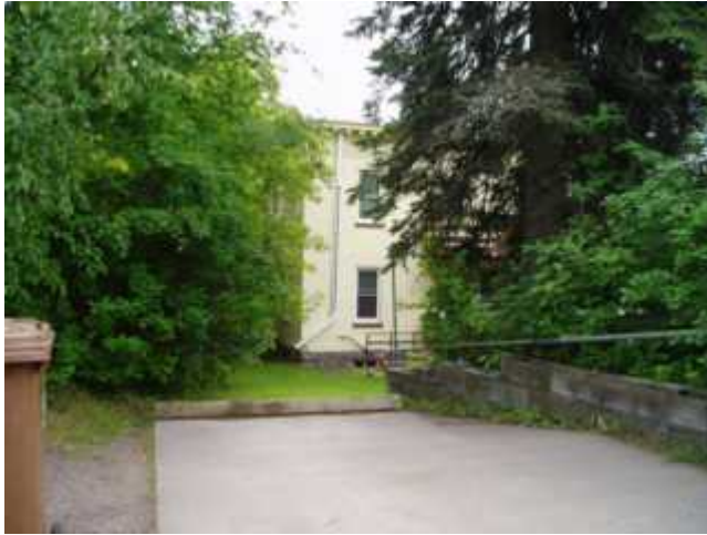
Figure 20. The Duluth, Minnesota, Weather Bureau Building in July 2004. Source: Jim Zandlo, State Climatologist for Minnesota.
