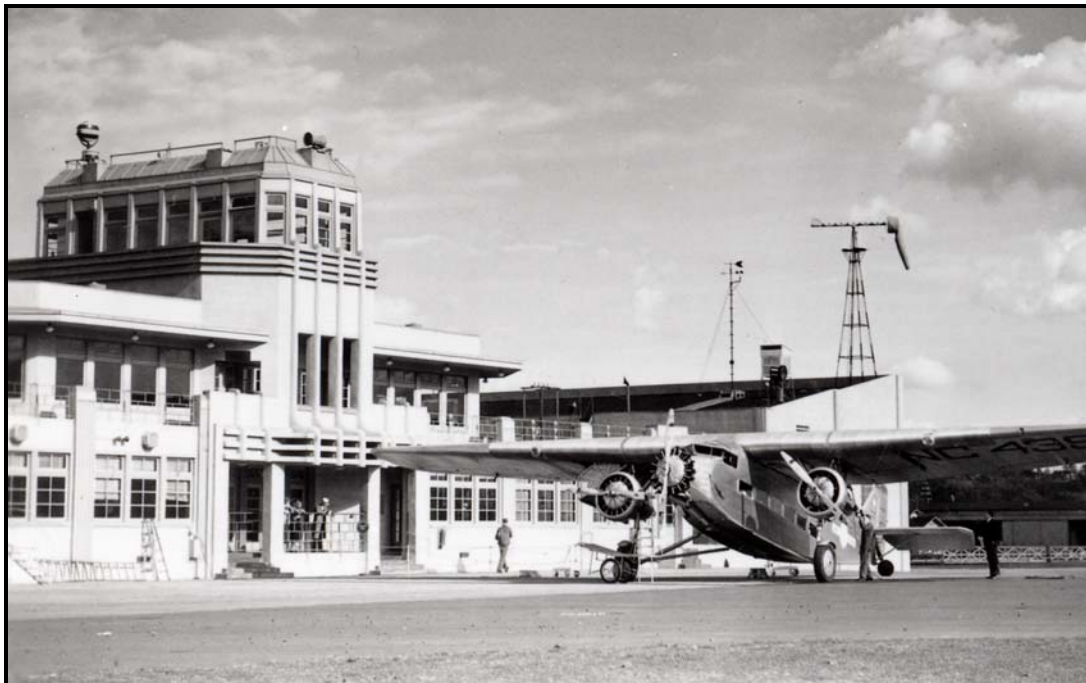
Figure 11. Administration Building for Swan Island Airport (circa 1930s) looking southeast. Weather Bureau instruments located on the southern roof of the building. From the Oregon Historical Society.
