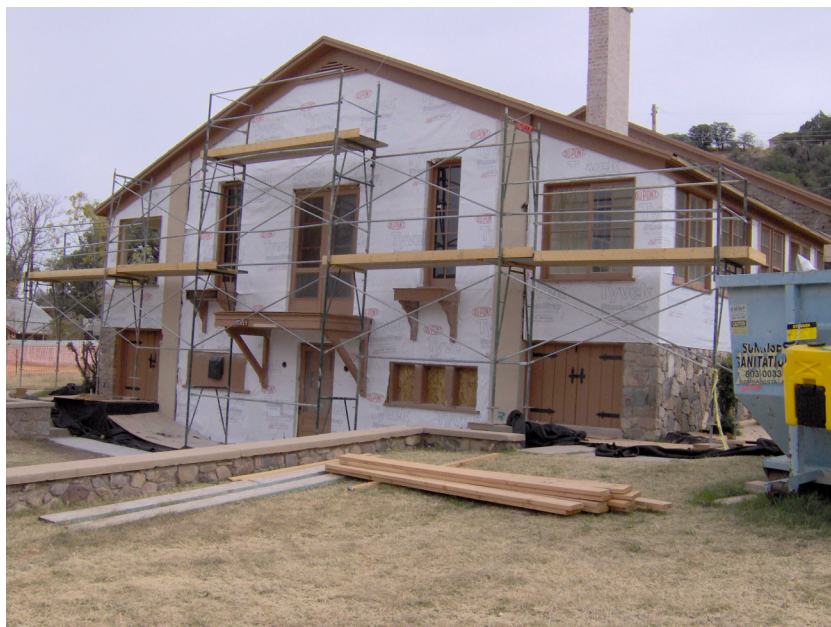
Figure 2. Carleton House Under Repair, the Second Hospital at Fort Huachuca, 2006 Source: Author
