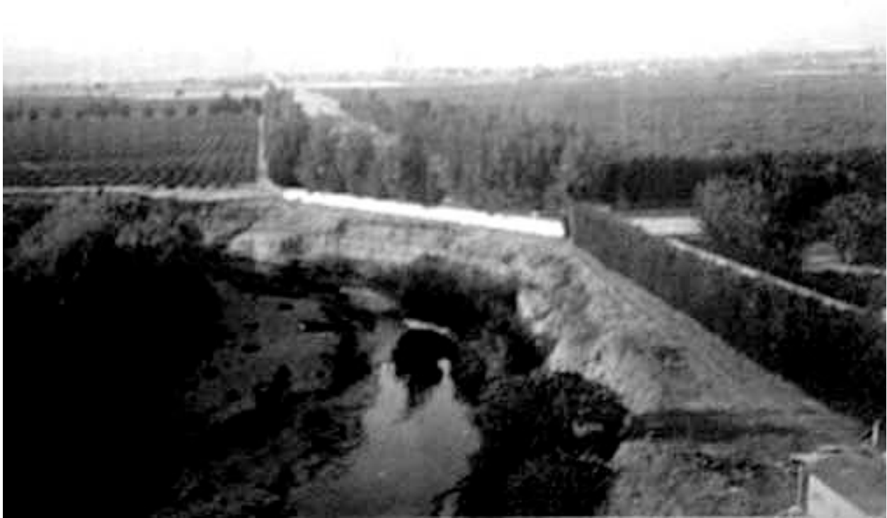
Figure 2. Looking North along Sonoma Creek Source: Depot Park Museum, Sonoma
