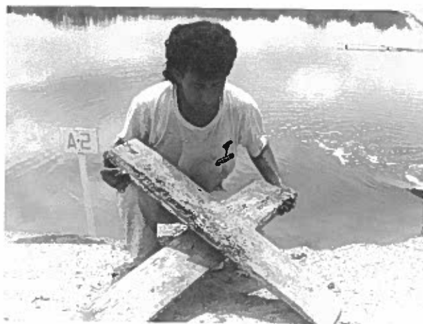
Plate 62. Rotten weir gate down board past the point of repair.
