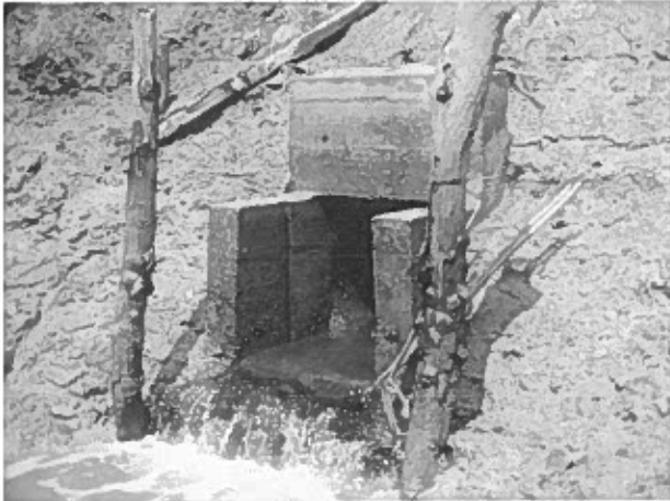
Plate 81. Effluent gate with simple culvert necessitates stopping harvest procedures when emptying bag net.
