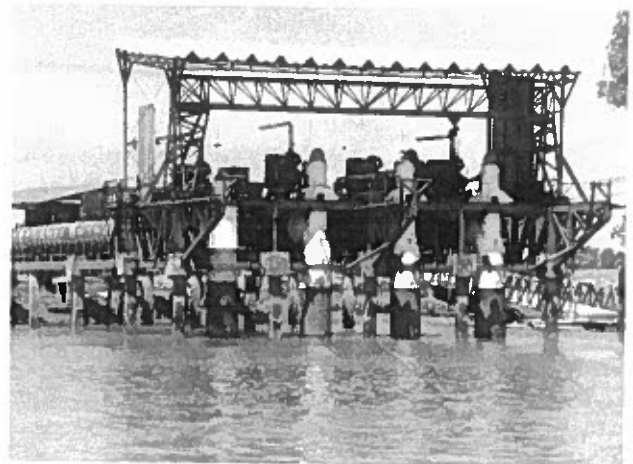
Plate 56. Typical central pump station for commercial farm.
