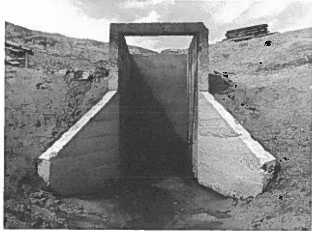
Plate 9. Pond weir gate scraped clean of filamentous algae and barnacles during disinfection. Note that weir boards are stacked in an orderly fashion.
