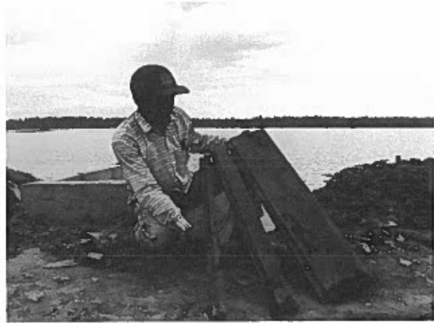
Plate 71. Various sizes of weir gate down boards. Notice varying widths, and tongued and grooved edges.
