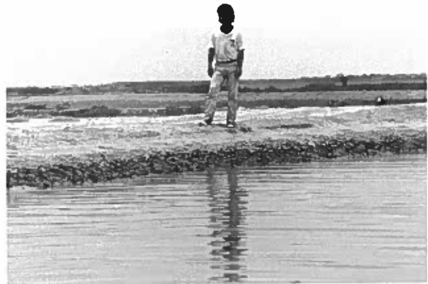
Plate 54. Crown of pond dike with 30 centimeters of "freeboard" above water level of pond.
