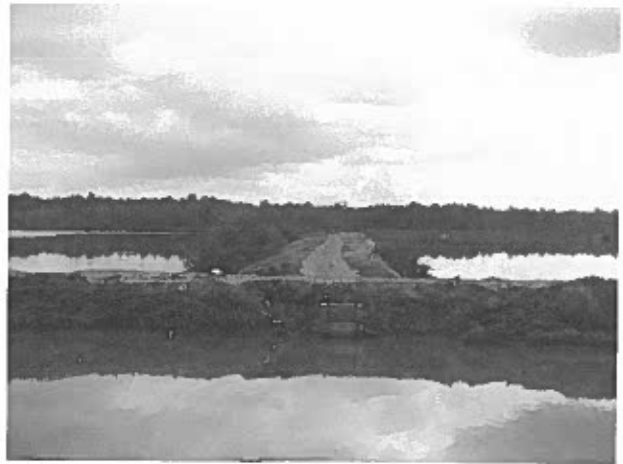
Plate 10. Entrance weir gate with restriction boards in place on the reservoir canal side of gate. If no board slides are on the reservoir side of gate, restriction boards should be nailed in place.
