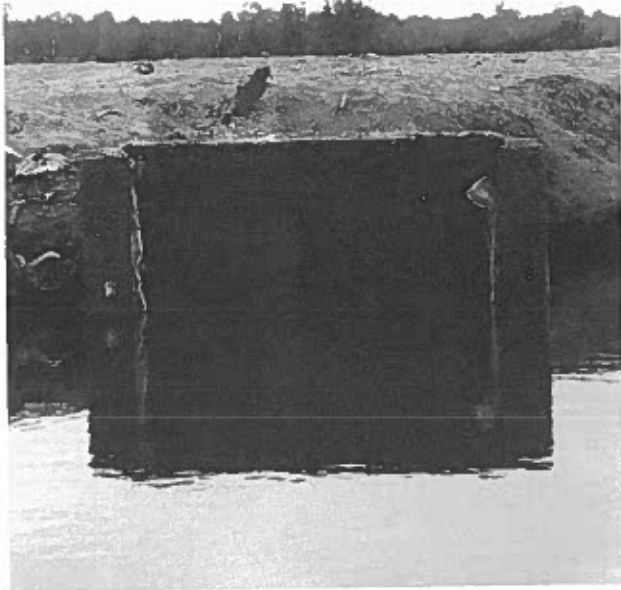
Plate 63. Empty feed bags positioned in weir gate slide channels to prevent water from filtering through borders.
