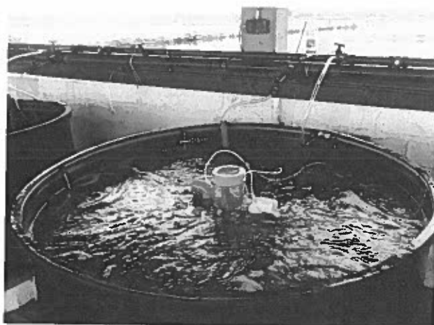
Plate 18. Air lift pumps functioning in filled acclimation tanks. Note: water circulation pattern is circular with pumps directed toward the tank wall.
