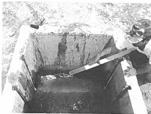
Plate 35. Approximately 20 cm of water draining over effluent down boards is allowed during transfer operation. The wooden pole and hand show water mark levels.
