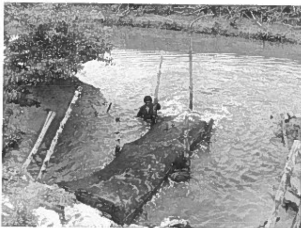
Plate 79. Harvest bag nets of 7 mm 2 netting firmly attached to effluent culvert.
