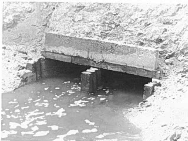
Plate 80. Effluent gate with divided culvert greatly facilitates harvesting procedures by eliminating the temporary suspension of harvest in order to empty bag.
