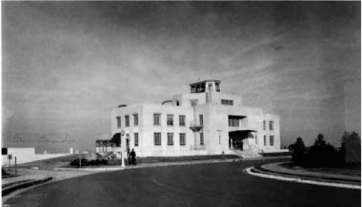
Figure 13. Administration Building 1942 Source: National Climatic Data Center
