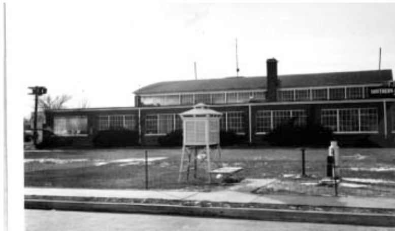
Figure 30. Instrument Shelter at the Airport in 1942 Source: National Climatic Data Center
