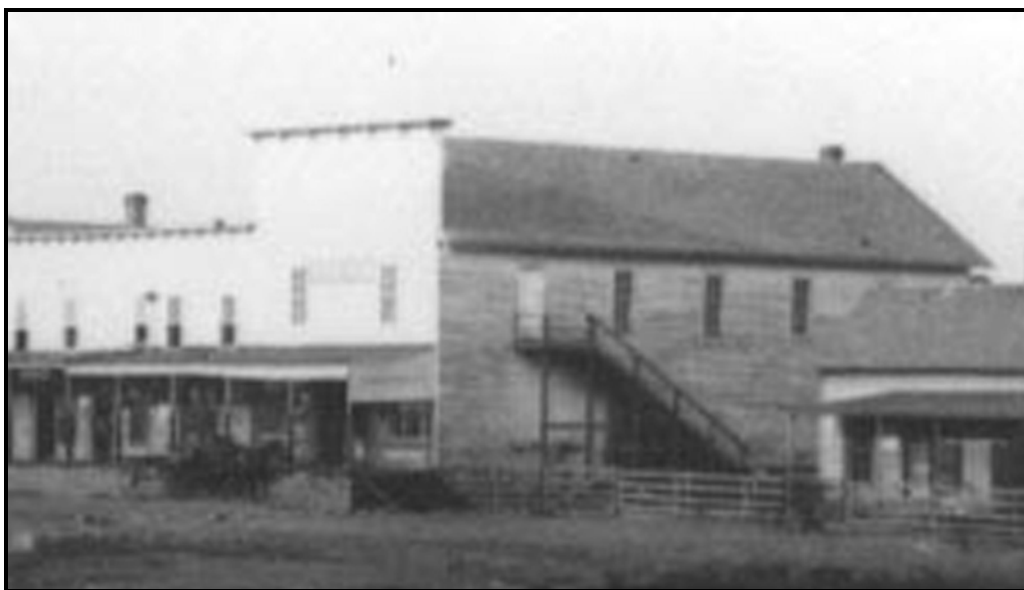
Figure 10. The Nash Building in the town of Fort Gibson that housed the Signal Service Office. View is generally north. Signal Service Office was located at the north corner and at the back of the building. From the Oklahoma Historical Society.
