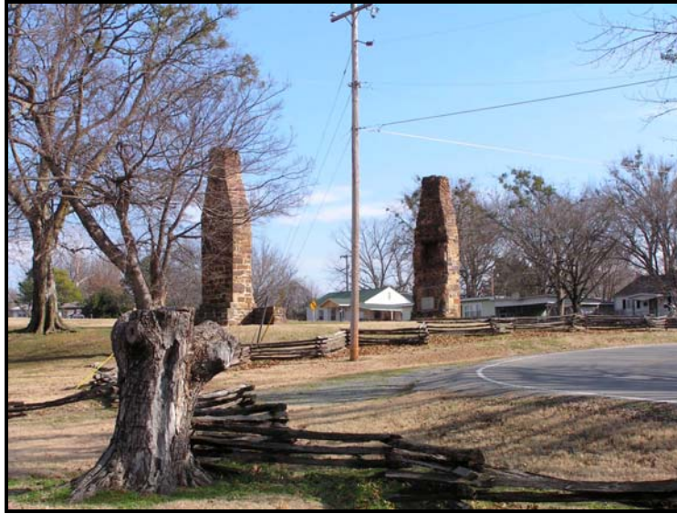
Figure 4. Location of the Fort Gibson surgeon quarters. View is towards the east-southeast. The hospital (1828 – 1870) was located to the right of the remains of the surgeon quarters in the photograph and in an area currently occupied by private residences shown in the photograph.
