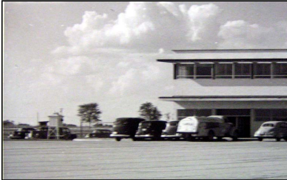
Figure 52. View of instrument shelter looking northwest (1952). From the LSUS Archives—Noel Memorial Library.
