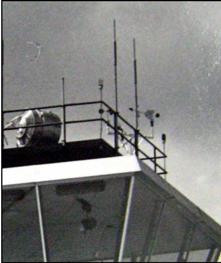
Figure 60. Enlargement of Figure 59 showing the wind instruments in 1952. View is northwest. From the LSUS Archives—Noel Memorial Library.
