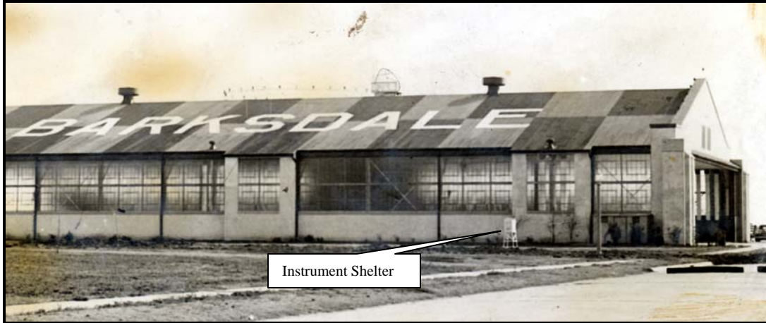
Figure 64. Hangar No. 9 and instrument shelter (circa 1930s). View is east northeast. Courtesy of 2 nd Bomb Wing History Office, Barksdale AFB, LA.
