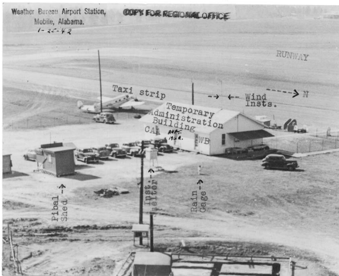
Figure 19. The temporary Administration Building on Bates Field, Mobile, Alabama, 25 January 1942. The location of the weather instruments can be clearly seen.
