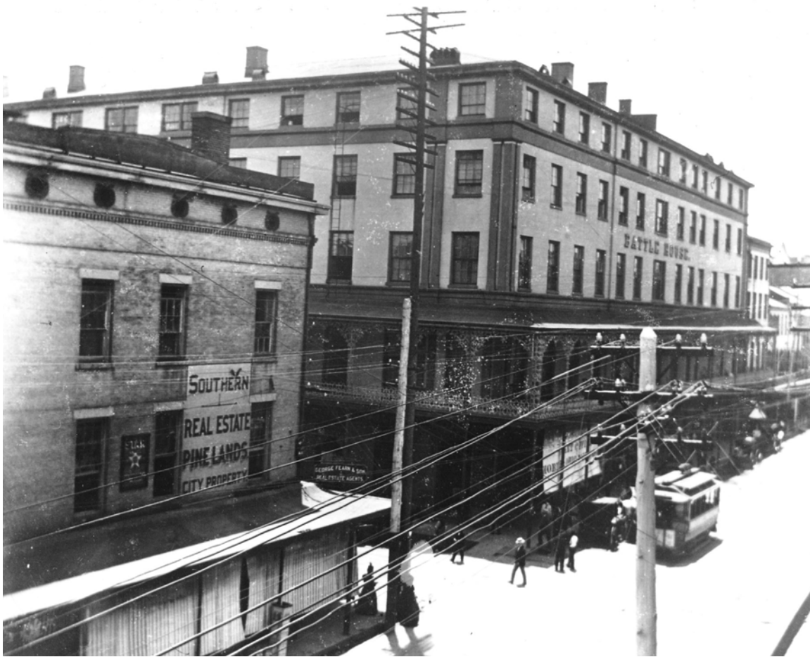
Figure 3. The Battle House in Mobile, Alabama, prior to it burning in 1905. View is looking southeast.
