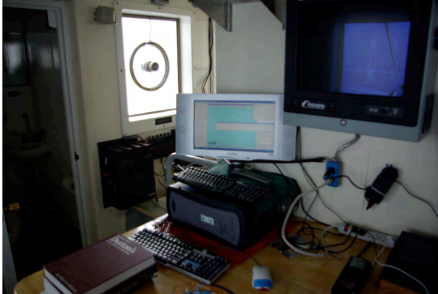
Figure 30 – Network Ground Station Installed On Ships Bridge.
