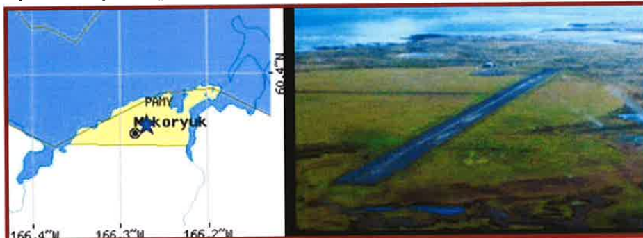
Figure 15. Location and Runway View of Mekoryuk Airport
