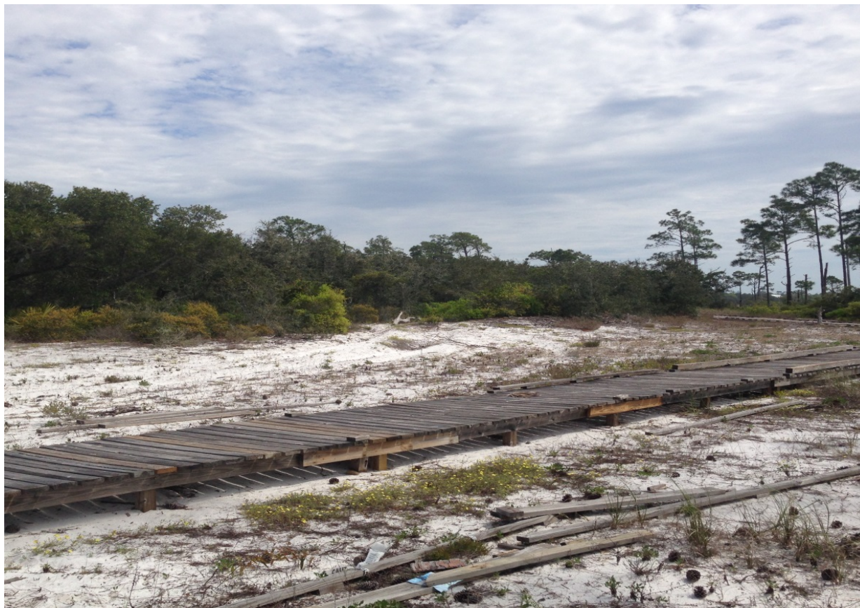
Figure 8-4. A portion of the existing Jeff Friend Trail boardwalk
