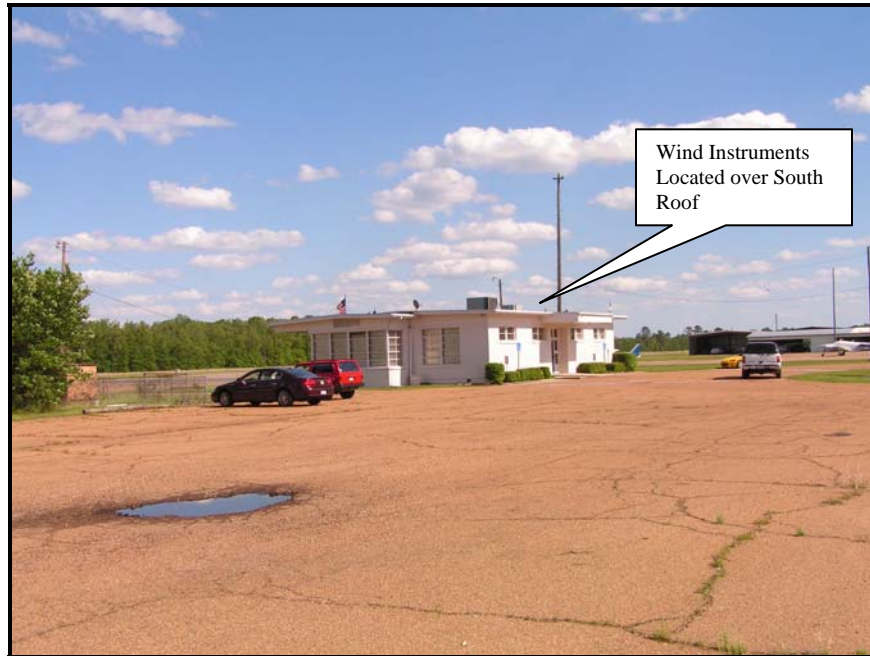
Figure 23. Administration Building at the Columbus-Lowndes County Airport. Airport officials stated this was the building that housed Southern Airways and the SAWRS in the early 1950s. View is southeast. Photograph by the author.
