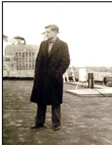
Figure 13. Tipping bucket and standard eight-inch rain gage on top of the Kimo Theatre Building (circa 1932). View is toward the south. Person in the picture was a Weather Bureau employee. From the files of the National Weather Service Forecast Office in Albuquerque, NM.
