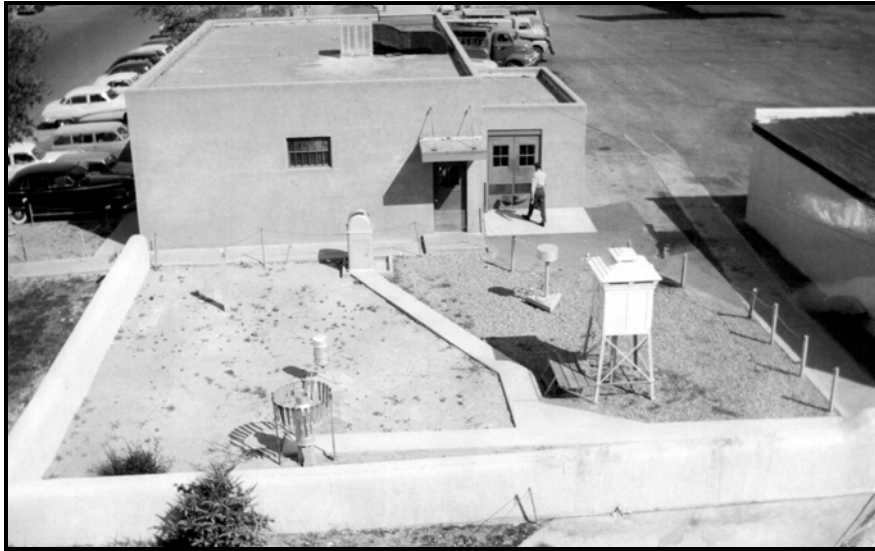
Figure 28. Exposure of the instrument shelter and rain gages on 22 September 1953 from the roof of the Administration Building. Note the new buildings immediately east and south of the weather instruments. On 23 June 1958, the instrument shelter and rain gages were moved to the roof of the TWA Express Building on the right side of the photograph. View is towards the east. From the official station history files at the National Climatic Data Center.
