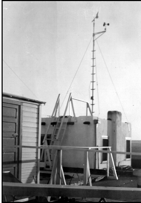
Figure 17. Close-up view of wind instruments on top of the TWA Office and Depot Building (circa 1933). Live chimney was located to the right of the wind instruments and extended slightly above the superstructure. View is south. From the official station history files at the National Climatic Data Center.
