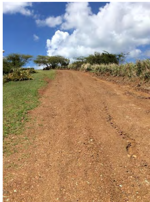
Figure 22. Pictures of existing conditions of the Fulladosa site before stabilization.
