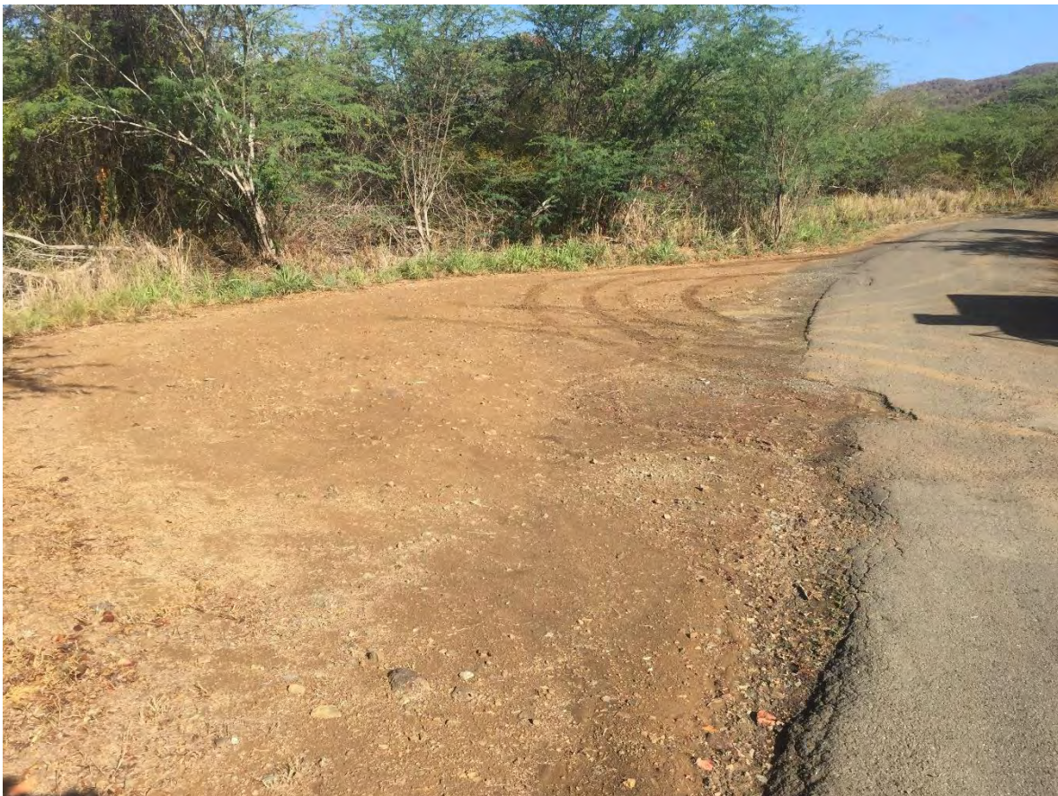
Figure 8. Turnaround site before stabilization.
