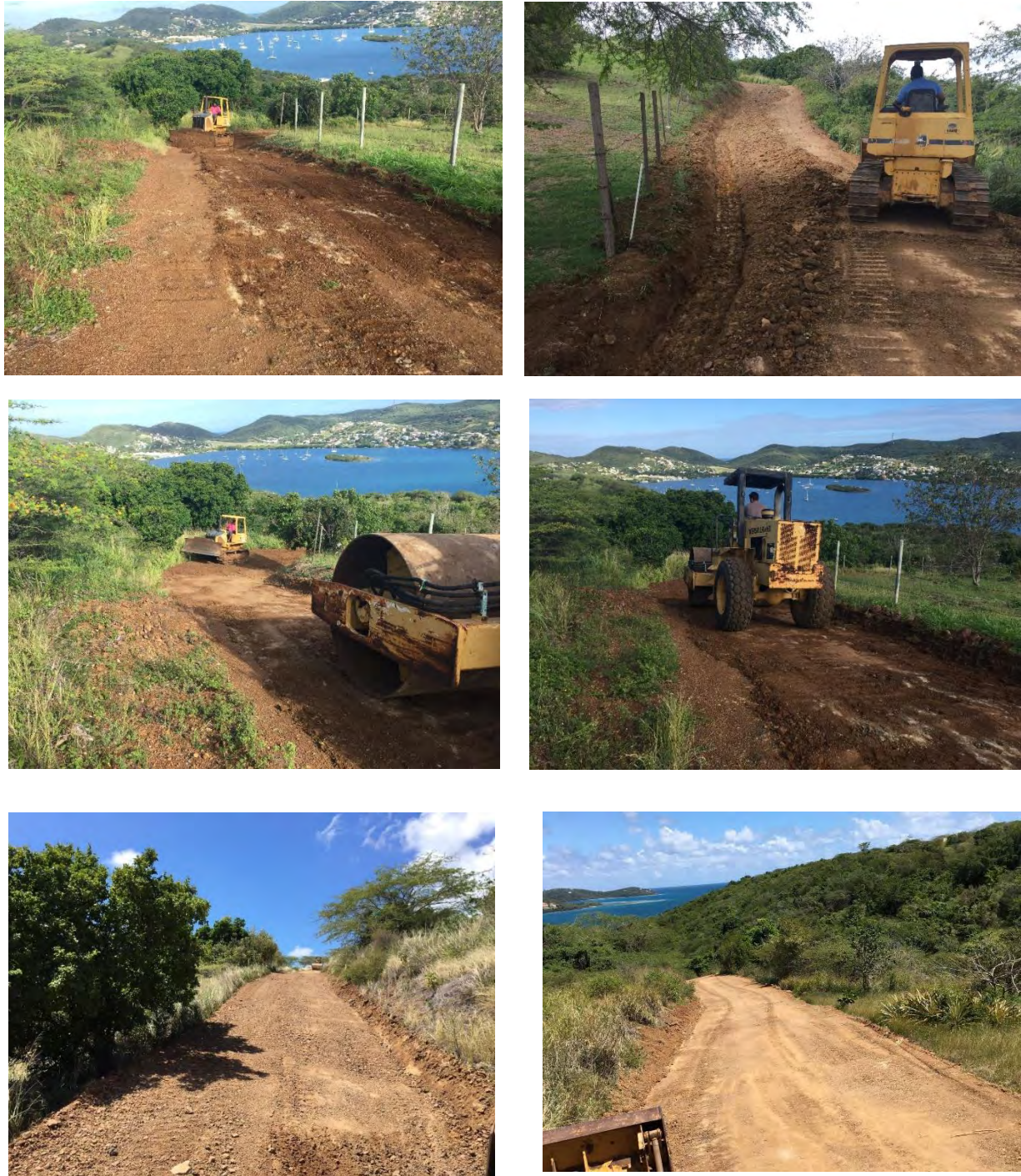
Figure 23-28. Pictures of regrading, compaction and stabilization process at the Fulladosa site.
