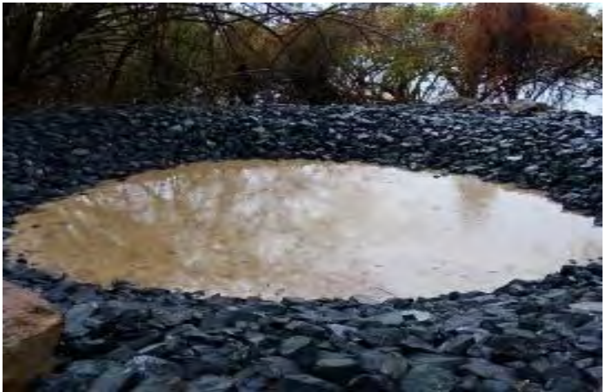
Figure 17. Sediment trap after a rain event of 2.5 inch.
