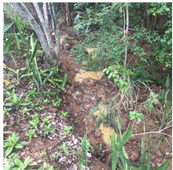
Figure 18. Pictures of existing conditions of the Fulladosa site before stabilization.
