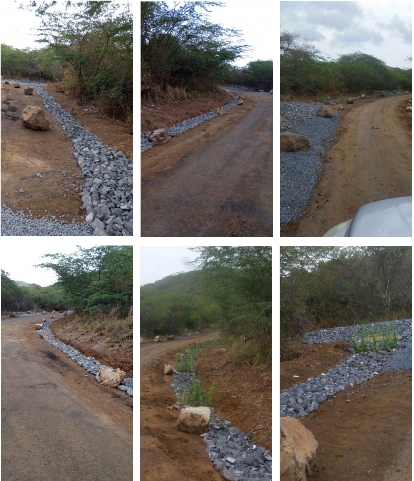
Figures 7. Pictures of some of the work completed.
