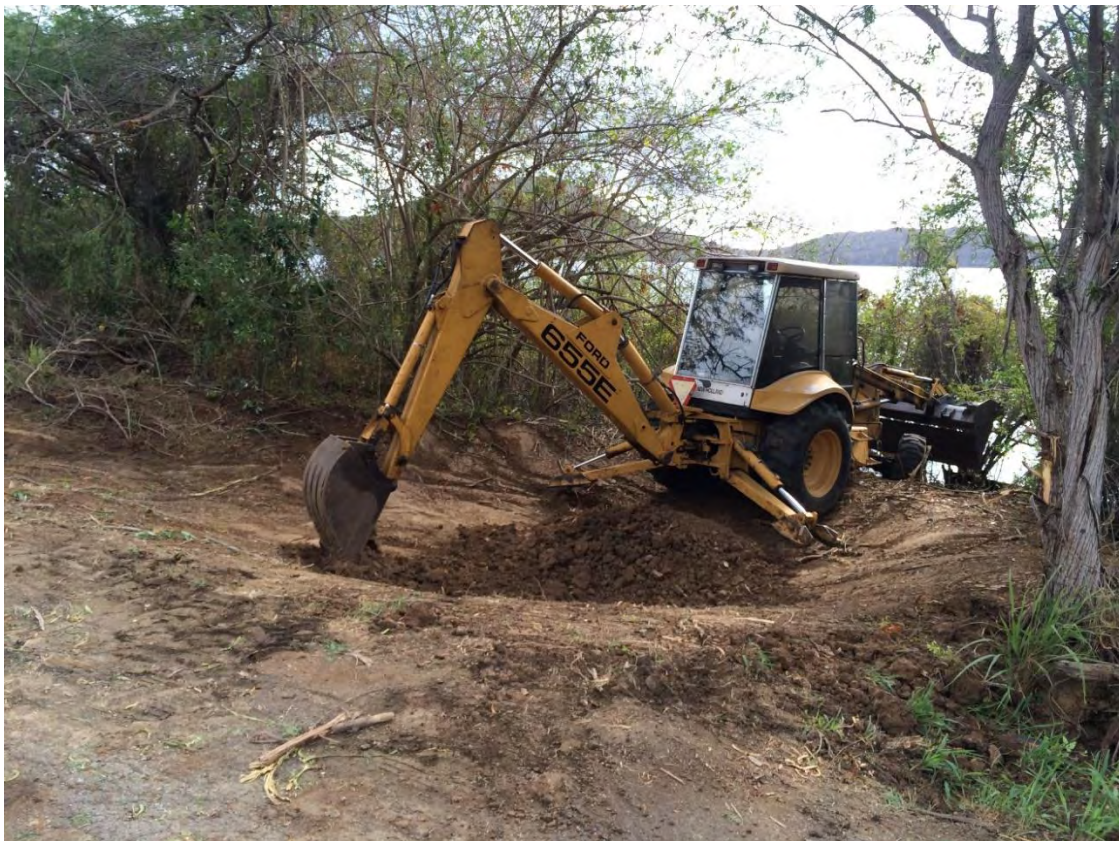
Figure 13. Construction of sediment traps process.
