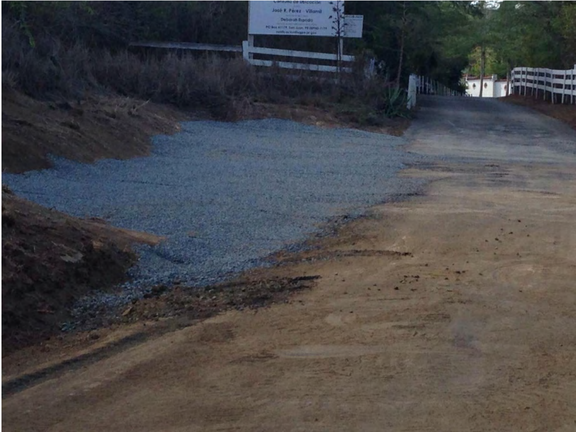
Figure 11. Turnaround site at Tamarindo during stabilization process.
