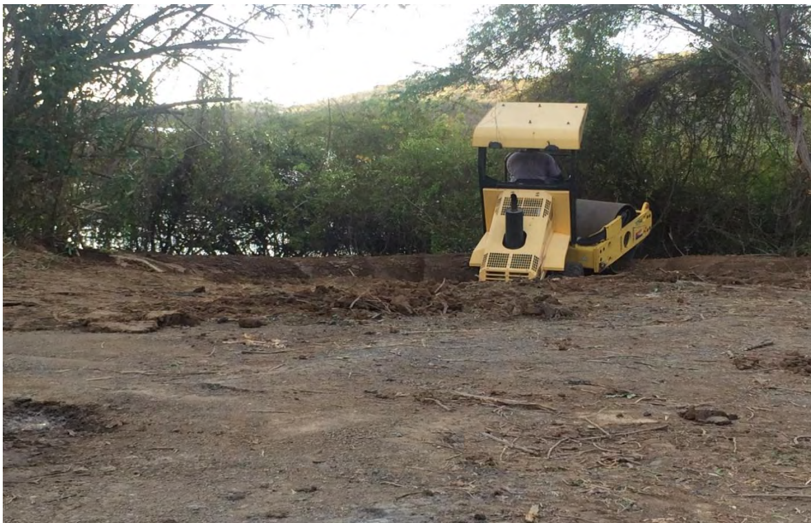
Figure 15. Sediment trap compaction of the berms process.
