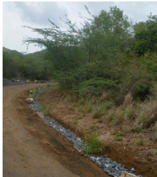
Figure 6. Stabilized culvert drainage.
