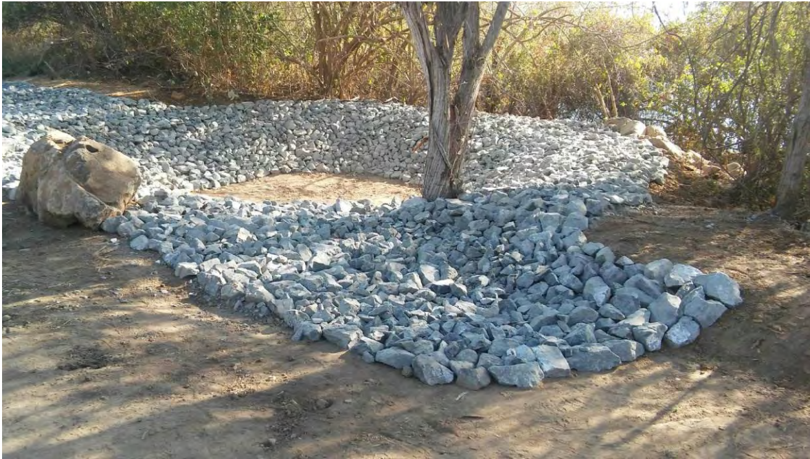
Figure 16. Sediment trap after stabilization.
