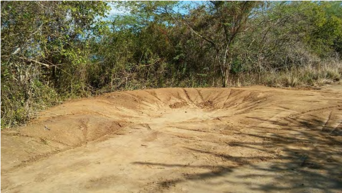
Figure 14. Sediment trap prior to be stabilized.
