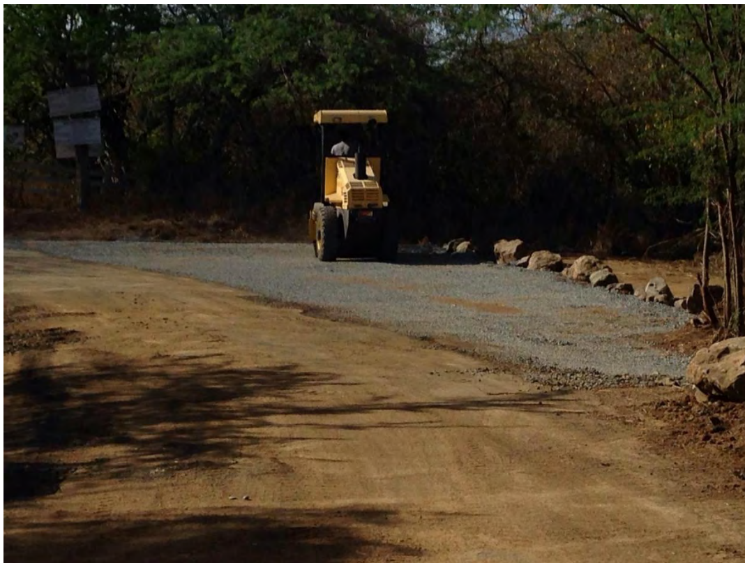
Figure 10. Turnaround site at Tamarindo during compaction process.
