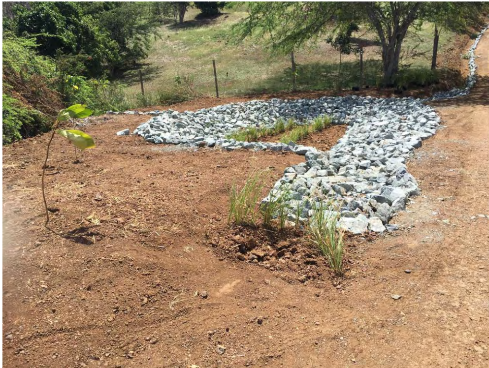
Figure 39-40. Pictures of second completed sediment trap at the Fulladosa site.
