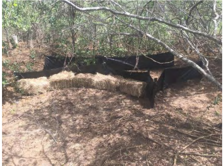
Figure 21. Example of temporary sediment control practices.
