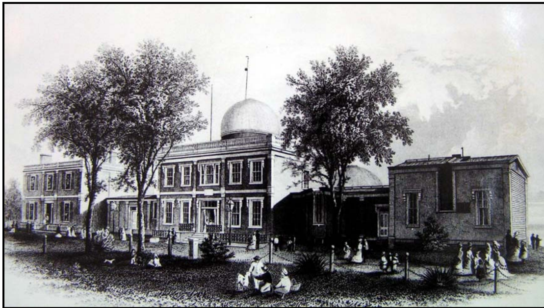
Figure 7. Naval Observatory buildings at Foggy Bottom (circa 1880). View is towards the southeast. The main building, in the center (with the dome), housed the operational barometer (located in the ground-floor room on the extreme right). The Superintendent’s house is on the extreme left of the engraving and housed the “standard” barometer. The transit circle house is located on the extreme right. Before May 1862, the dry bulb and wet bulb thermometers were hung on the north walls of the building connecting the main
