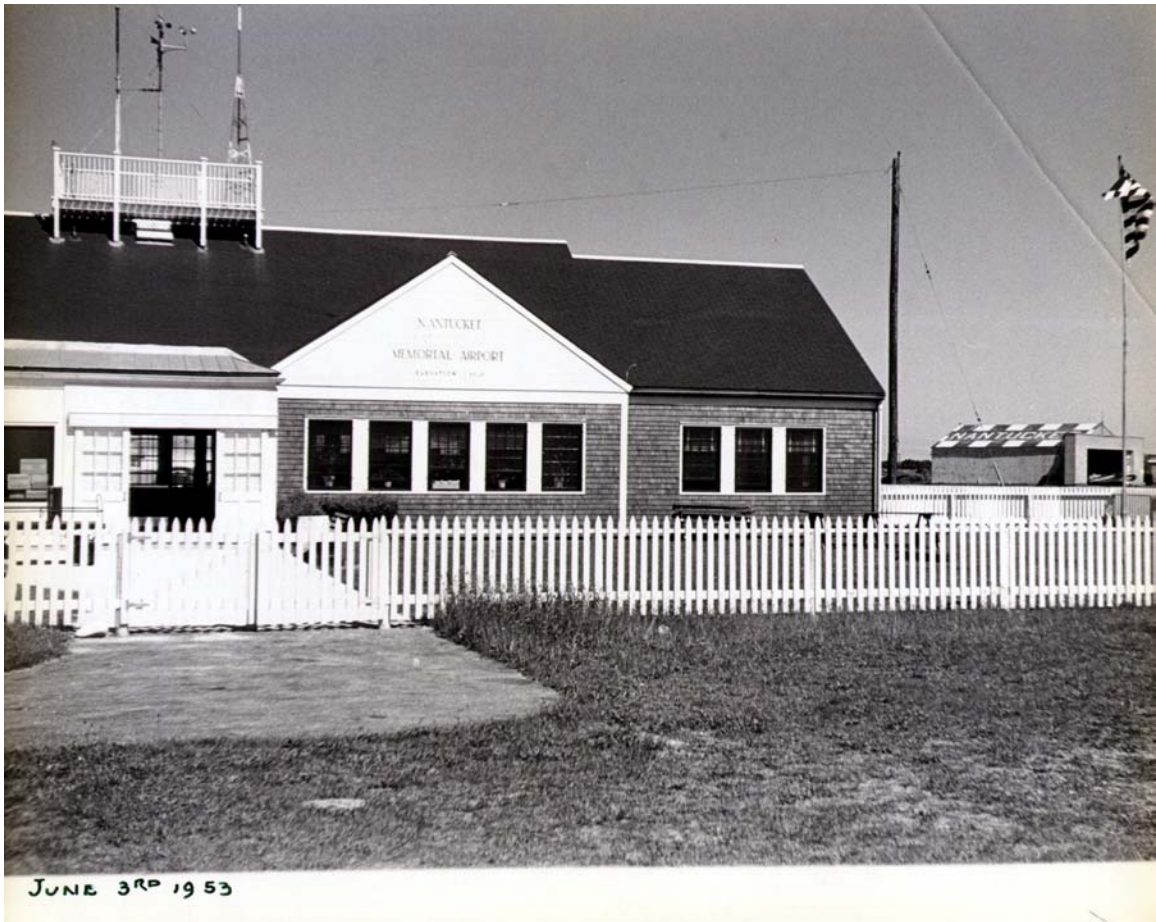
Figure 20. The Nantucket, Massachusetts, Memorial Airport terminal building as of June 3, 1953. The wind instruments are visible on the roof. Photograph from the Nantucket Historical Association (P21023).
