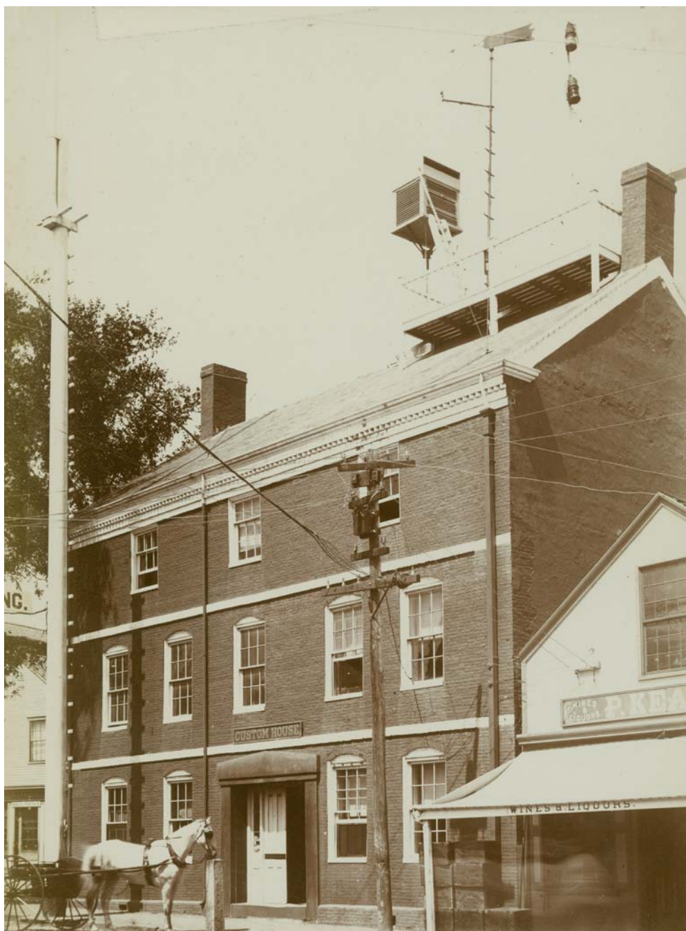
Figure 7. The Pacific Club Building (Custom House) in Nantucket, Massachusetts, circa 1900. Notice instrument shelter and wind instruments on roof platform. Also notice that electricity has come to the building. Photograph from the Nantucket Historic Association (P15479).
