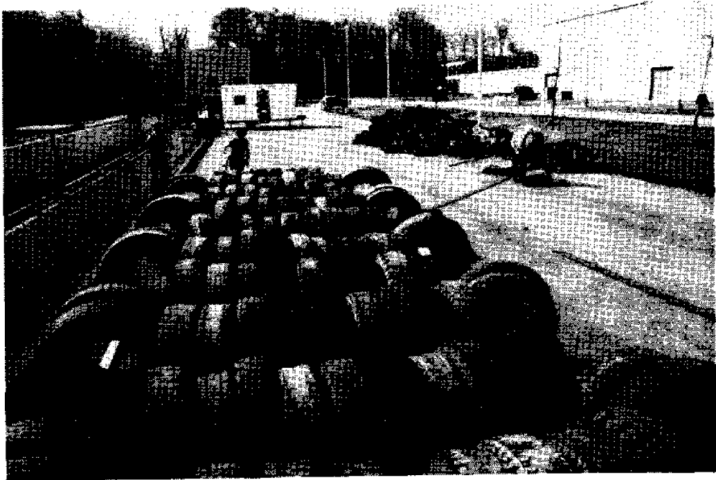
Fig. 7 Tires are in Position, Ready to be Tied
