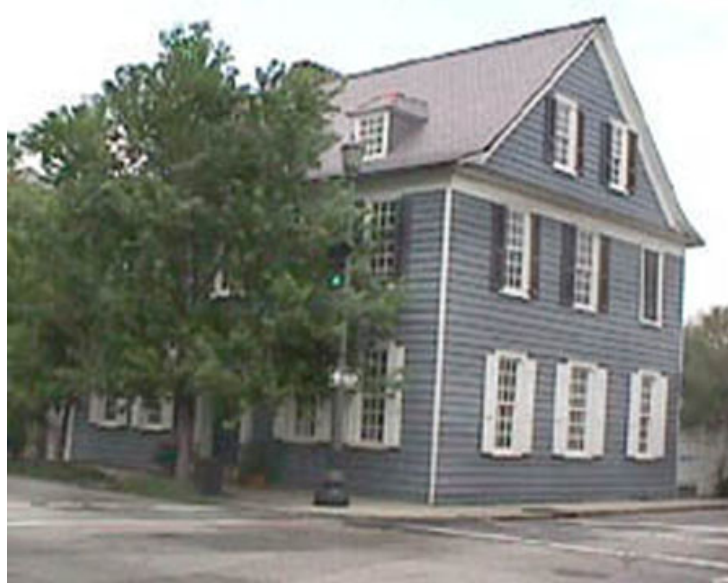
Figure 2. The home of Dr. John Lining, located at 106 Broad Street, Charleston, South Carolina, circa 2000. House faces south. Source: Charleston County Public Library
