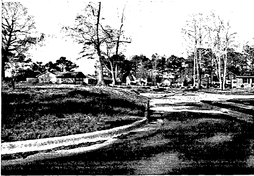
Curbs and gutters channel street storm water into drains in this West Havelock subdivision.
