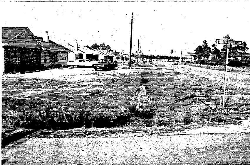
Open ditches and no curbs and gutters in this area of east Havelock retain some water days following rain showers.
