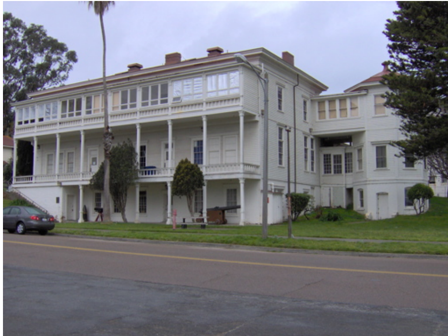
Figure 3. Post Hospital in 2005 as viewed from the east
