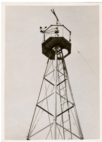
Figure 11. Wind Instrument Tower, Roof Federal Building, San Francisco Source: With Permission of the San Francisco Public Library
