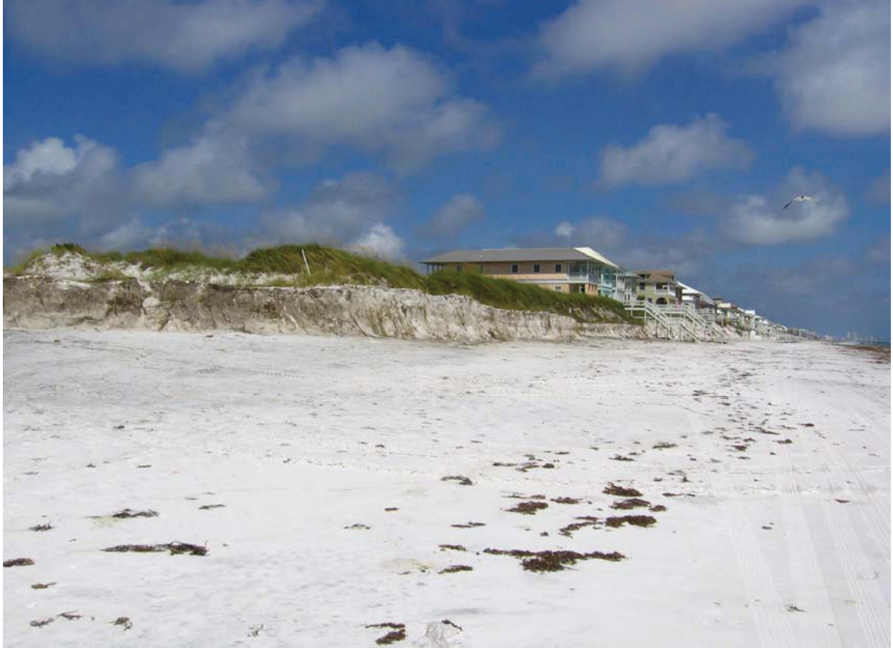
Figure 3. An example of coastal erosion at Carillon Beach, post-Hurricane Dennis.
