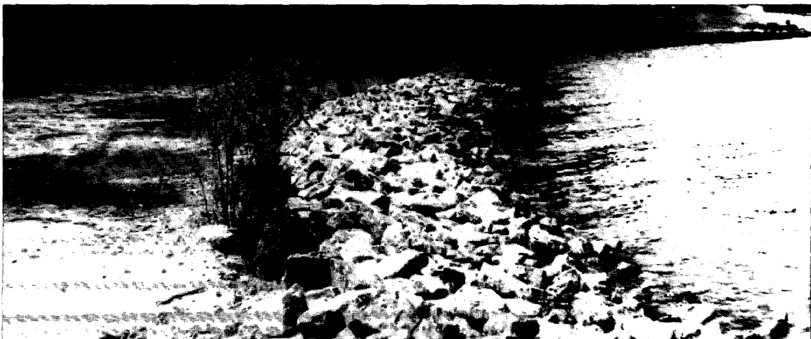
Figure 15 — Concrete seawall (top). Figure 16B (bottom) small riprap revetment. Figure 16A (middle) riprap revetment.
