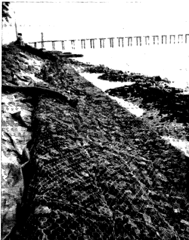
Figure 22 – Gabion revetment.
