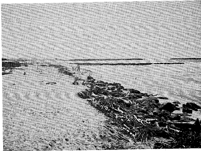
Downcoast view of groin no. 1, San Buenaventura State Beach, Mar. 15, 1978
