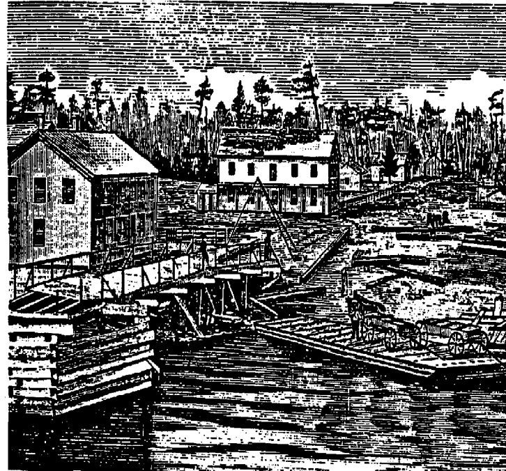
View of Alpena - 1865 - Constructing first bridge.
