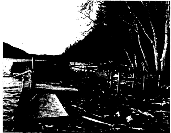
Debris-laden floods relocated these cabins in the January 1983 Presidentially-declared flood disaster in the Blue Canyon area on Lake Whatcom.
